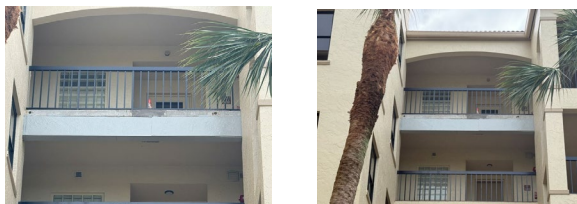
D Building fifth-floor waterproofing • September 25, 202
