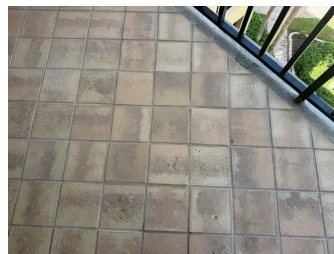
Completed Tile Repair in front of D-502
