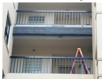
Paper-backed lath installed 10/5/26
