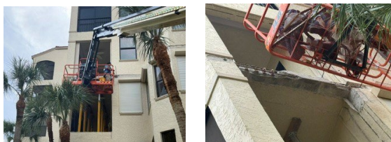
PT Pros Working on PT Cables F-205/F-305
