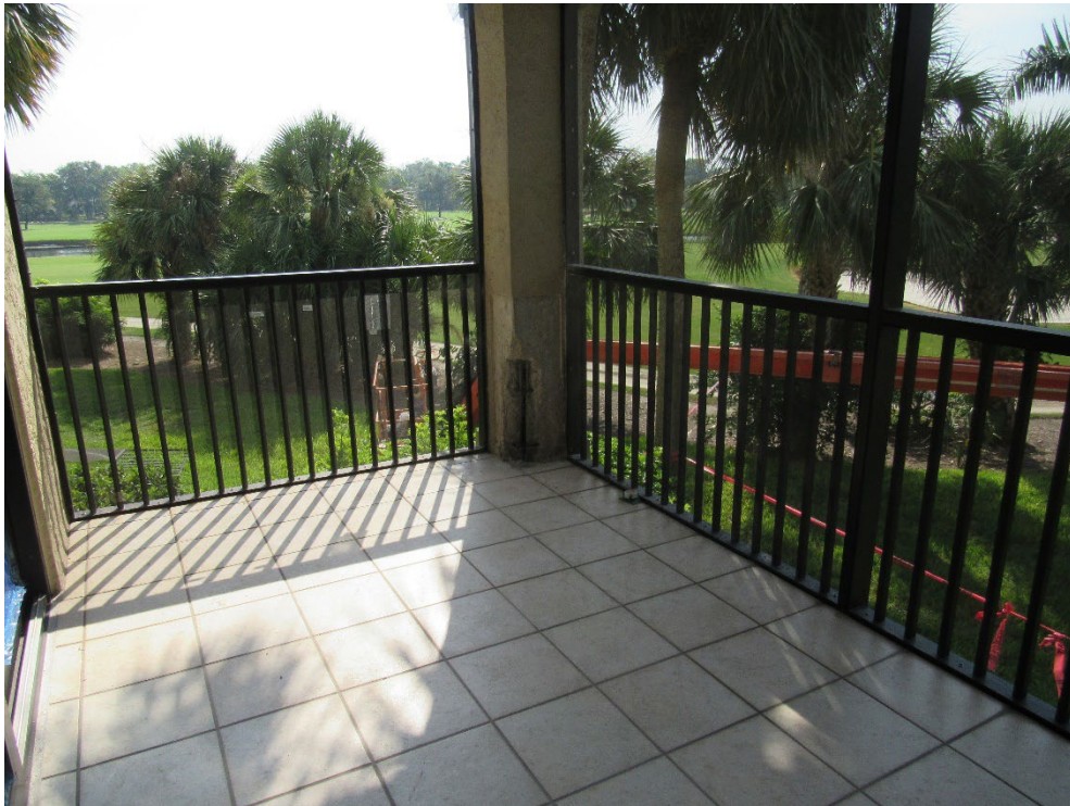
Overview of unit F103 balcony.
