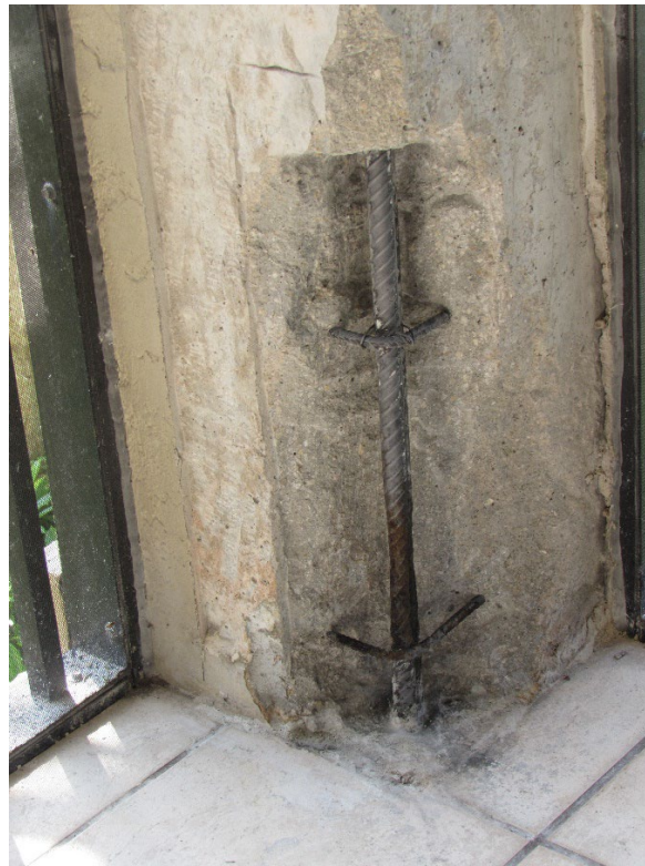
View of ongoing concrete restoration procedure at balcony column.
