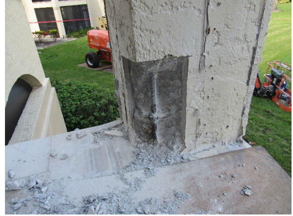
104 column repairs
