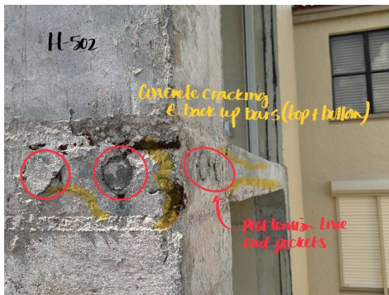
PT cables at column
