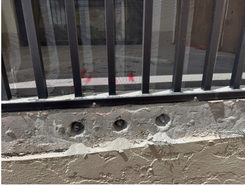
Unit F-304 – 3 band line cables identified in the suspected dead-end location.
