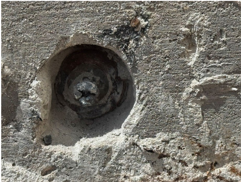
Unit F-304 – 3 band line cables identified in the suspected dead-end location.
