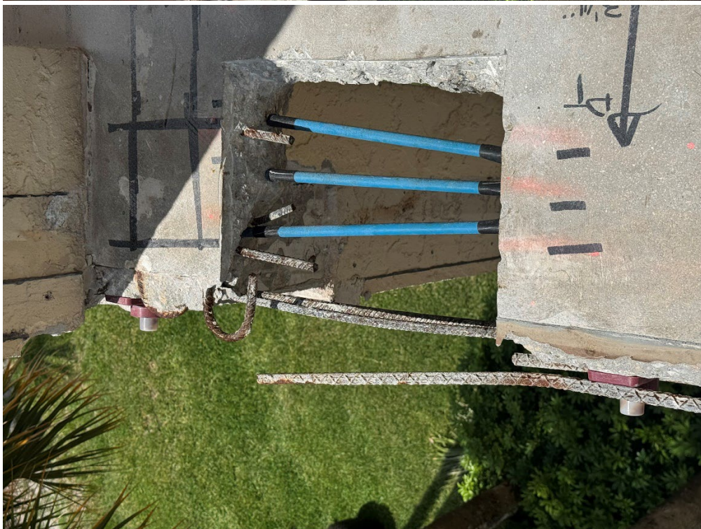
Unit F-303 – Full cable replacements completed for the 3 uniform cables emanating from the column.
