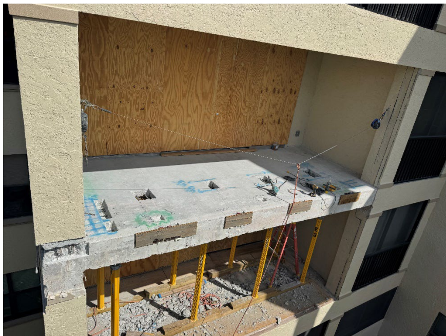
Full view of Unit F-301 balcony deck, showing completed uniform cable repairs.
