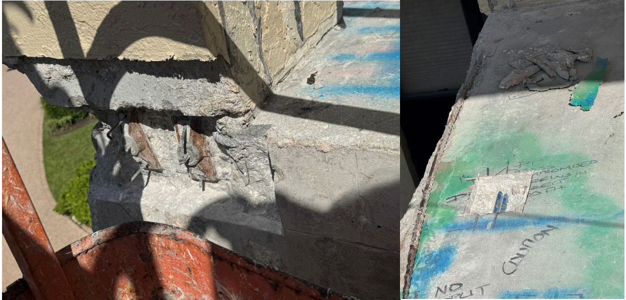
Remaining uniform cables requiring full cable replacement, showing clearance between the cables and proximity to band line cables, Unit F-301.
