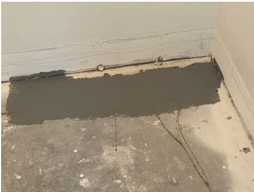
Observed completed interior structural slab crack repair.
