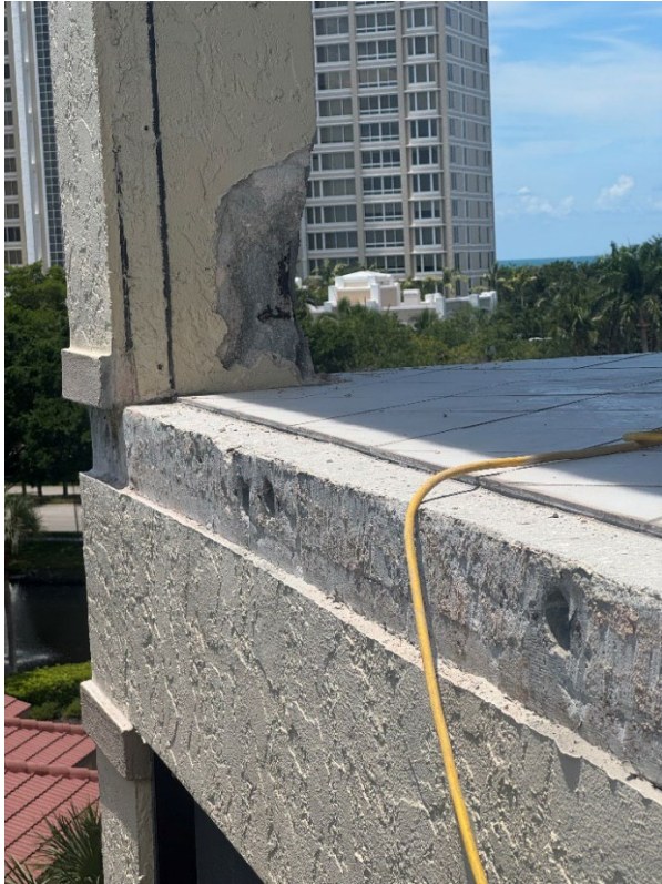
Left side slab edge repair:
