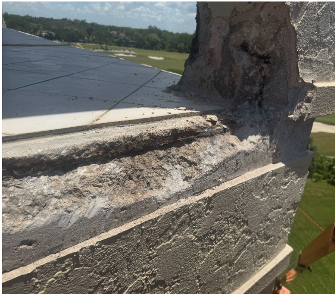
Left side slab edge repair:
