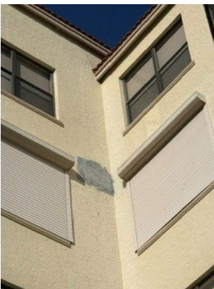
H Bldg. 5 th floor 3 stack additional Stucco repairs
