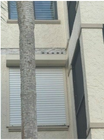
F Bldg. 5 Stack PT pockets
