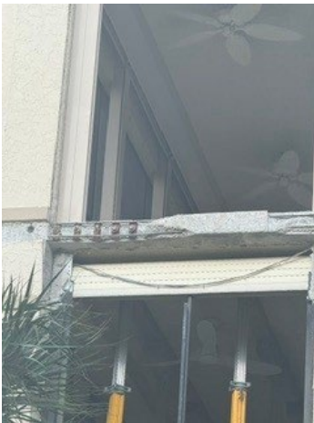
F Bldg. 5 stack pt pockets and concrete repairs
