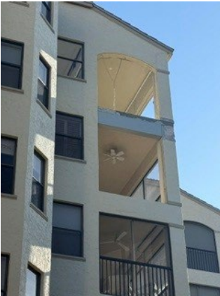
H Bldg. 1 Stack
