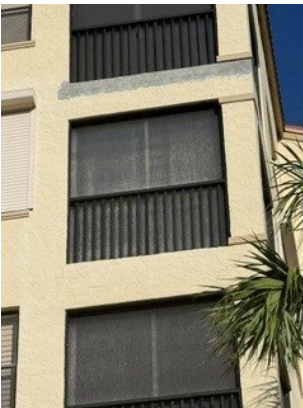
H Bldg. 5 th floor 3 stack stucco Repair
