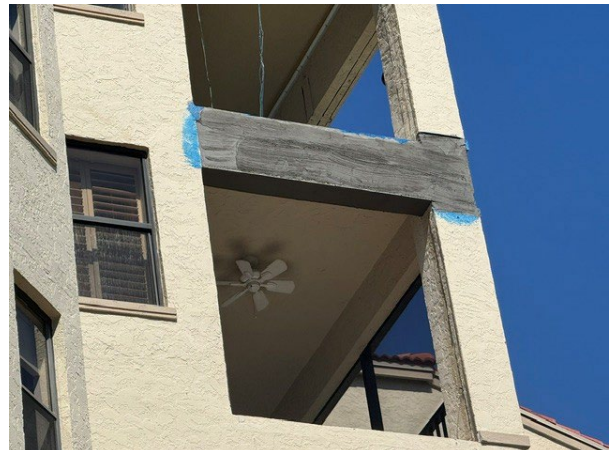
H-401 Scratch coat of stucco on header 925-26
