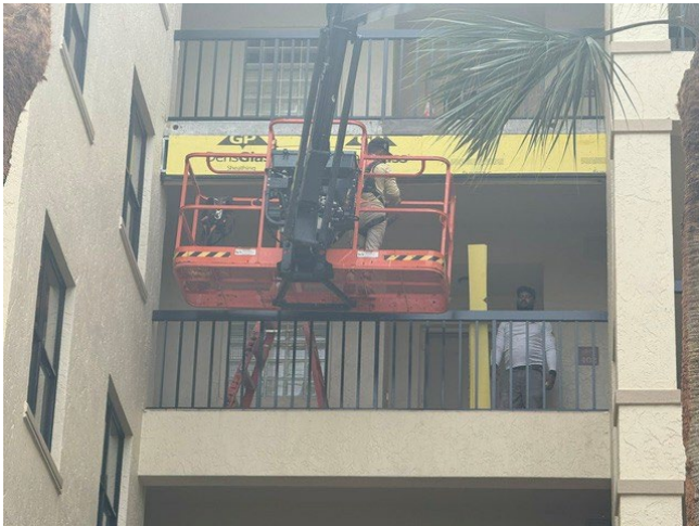
D Building fifth-floor sheeting • September 21, 2026
