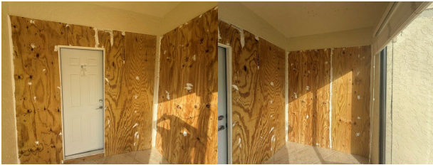
Temporary walls on F-204's small lanai
