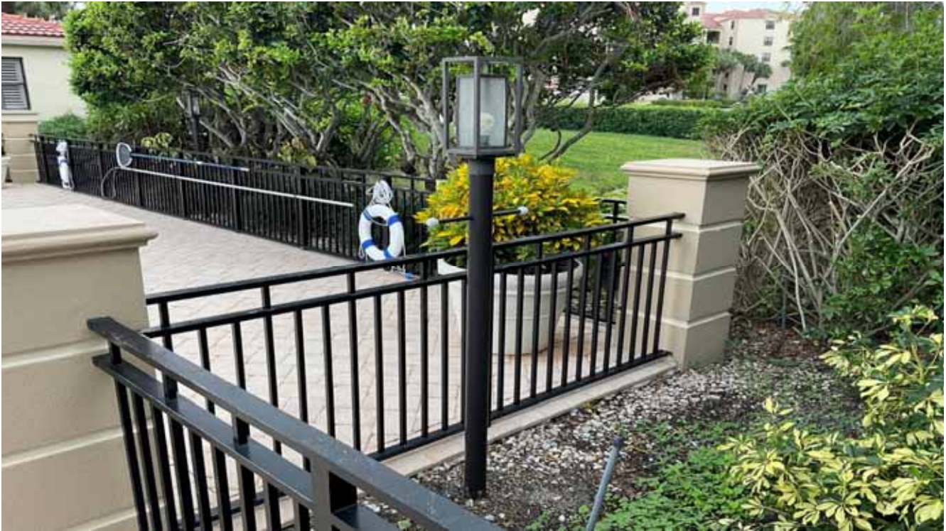
Light Pole & Fixture - Pool Area
