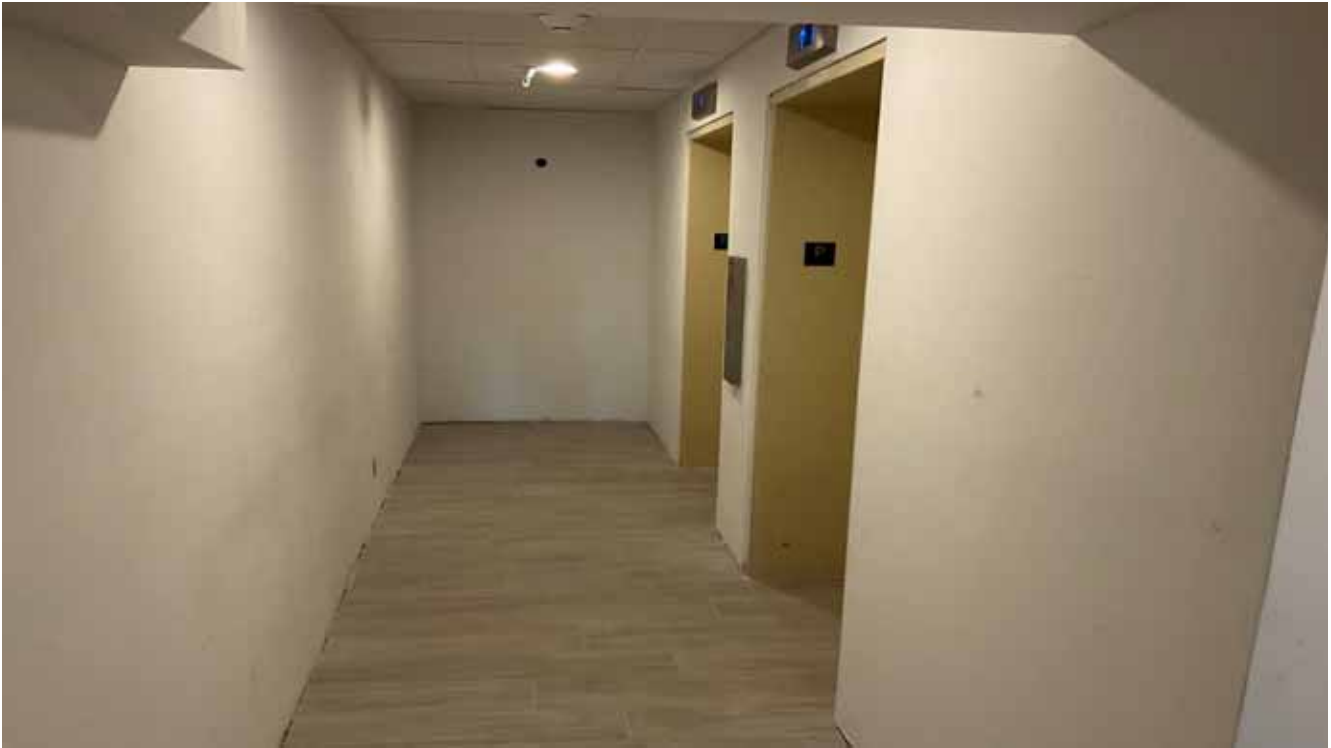
Building F Elevator Lobby - Garage
