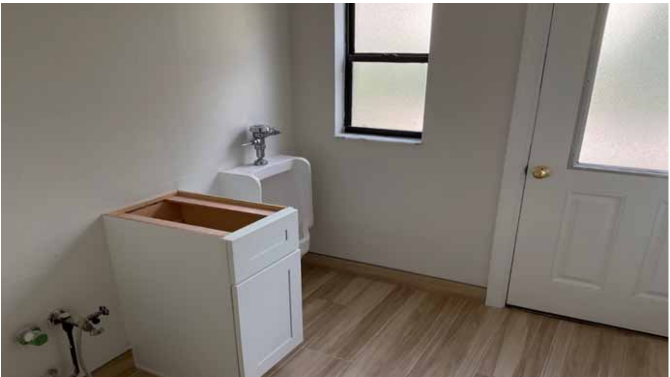
Clubhouse Restroom, Men's
