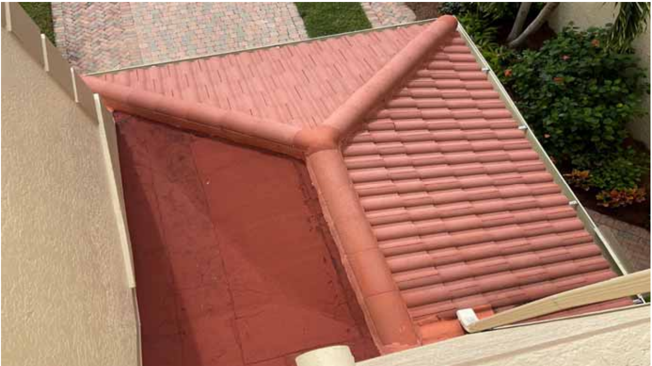
Building C Roof - Lower
