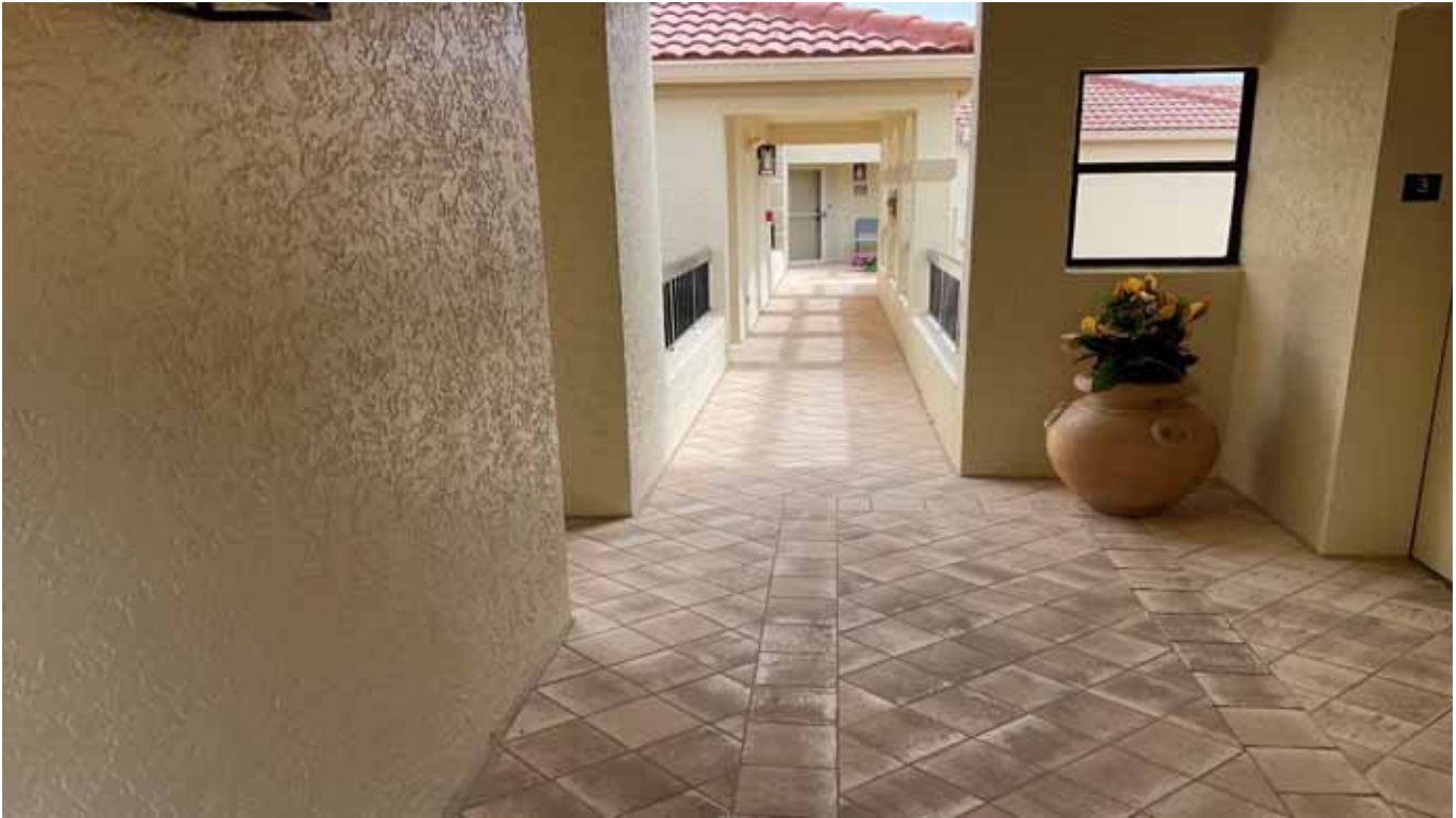
Building C Walkway - Upper Floor
