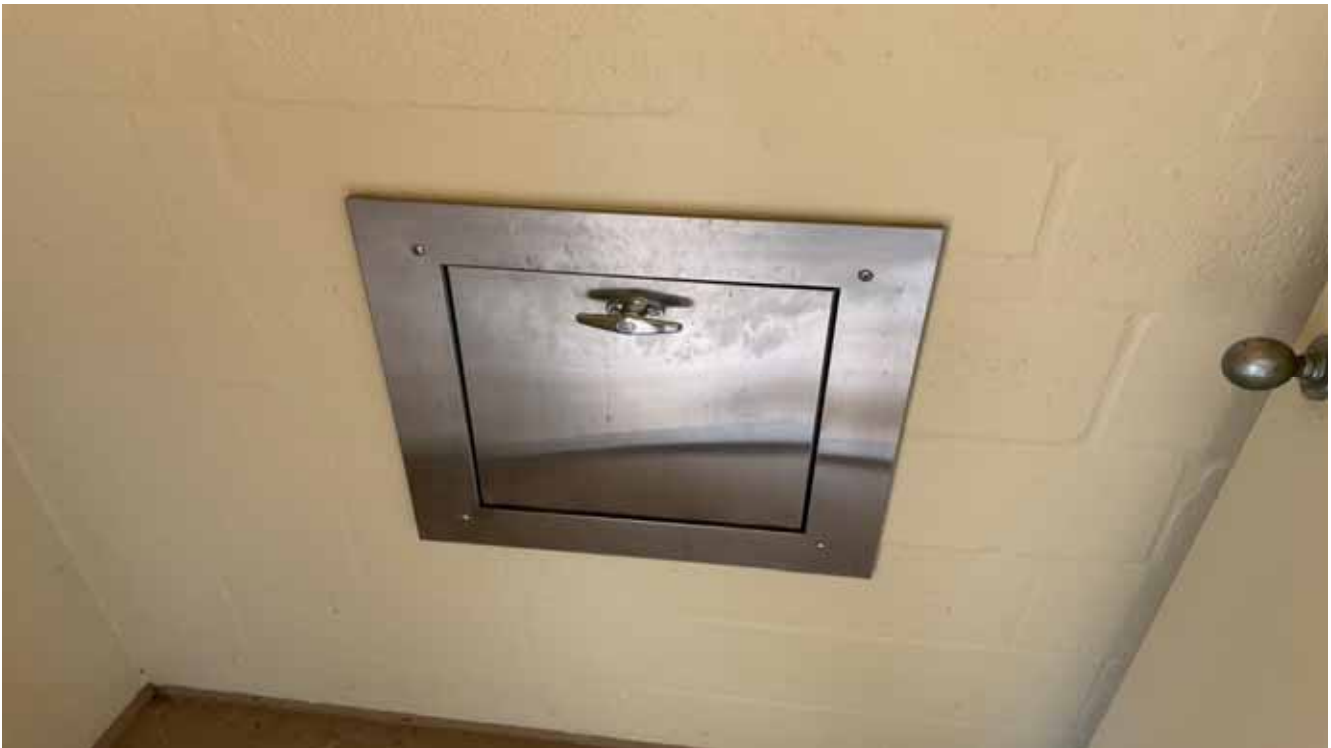
Building E Trash Chute Door
