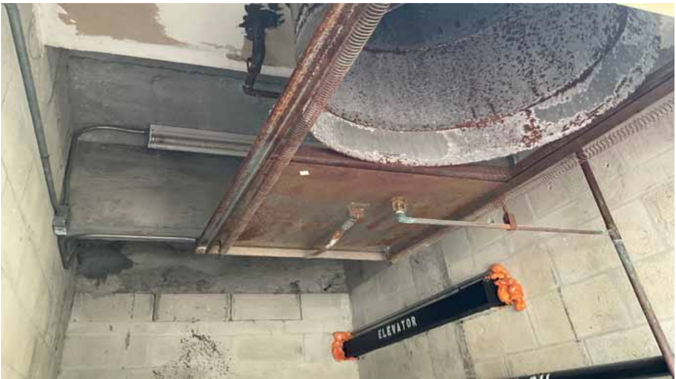
Building E Trash Chute Guillotine
