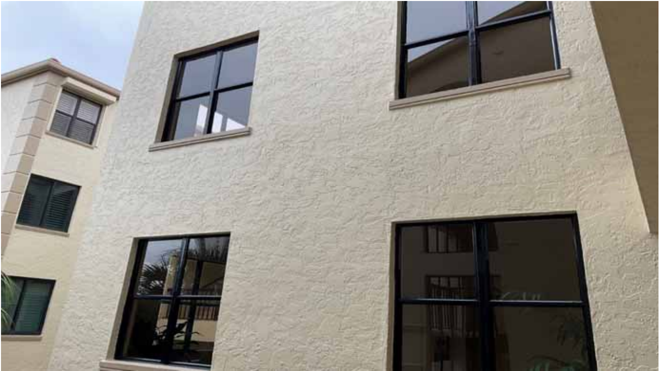
Building F Elevator Lobby Windows - Upper Floor
