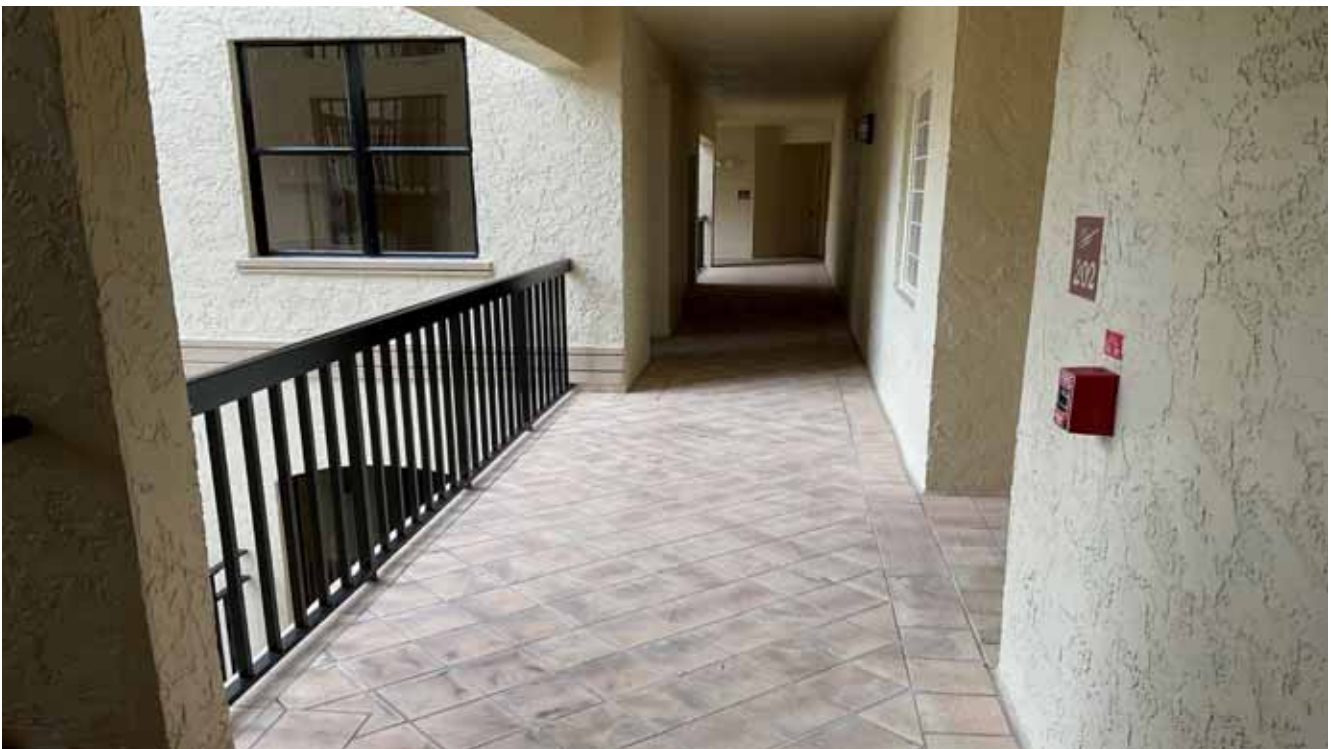
Building H Walkway - Upper Floor
