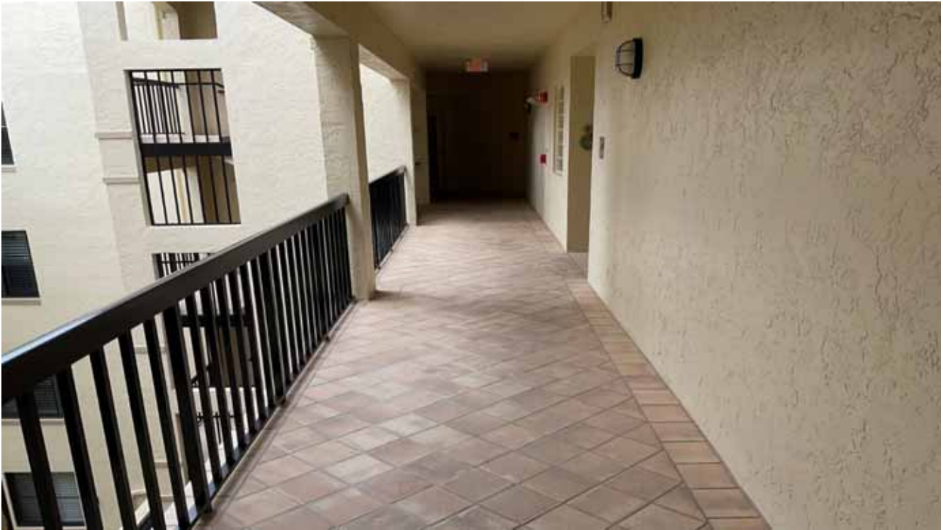
Building D Walkway - Upper Floor
