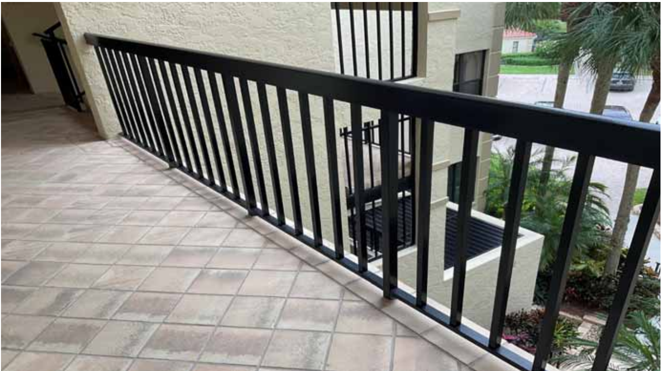
Building F Walkway - Upper Floor
