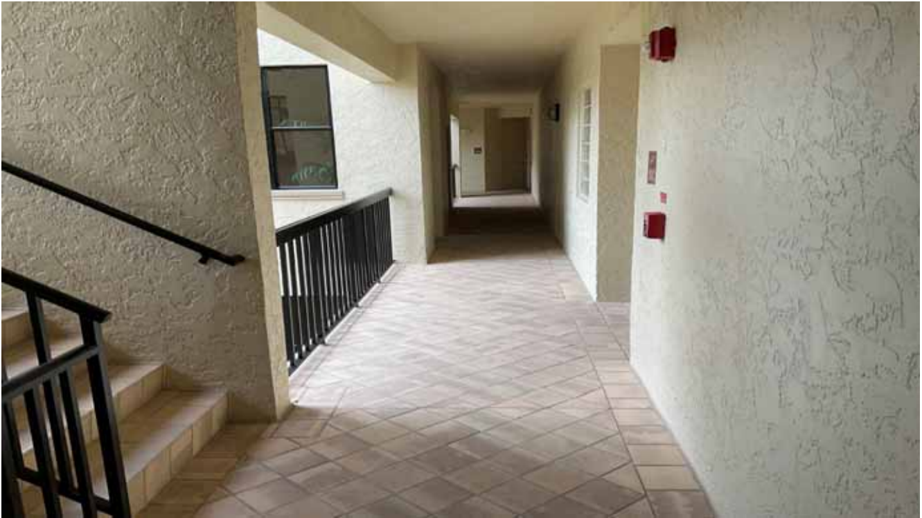
Building F Walkway Railing
