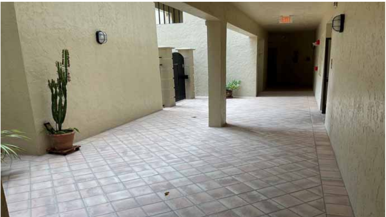
Building D Walkway - First Floor
