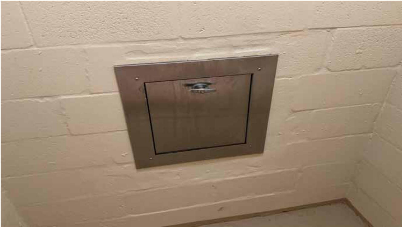
Building F Trash Chute Door
