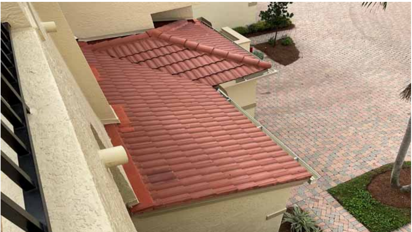
Building E Roof - Lower
