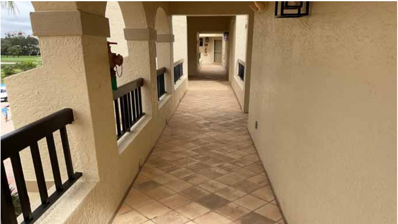
Building E Walkway - Upper Floor
