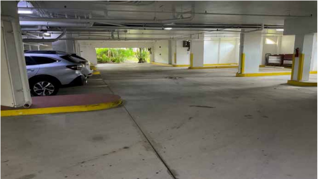
Building H Garage
