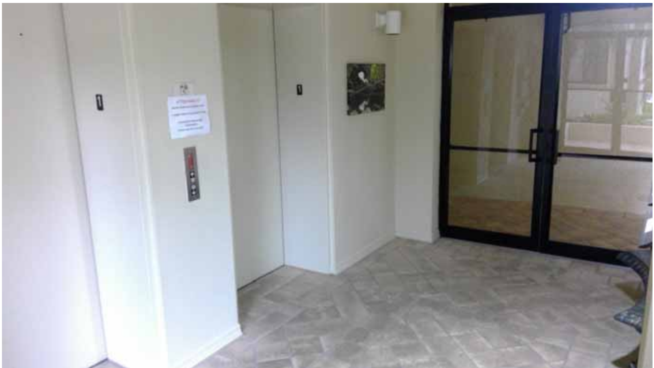
Building H Elevator Lobby - First Floor
