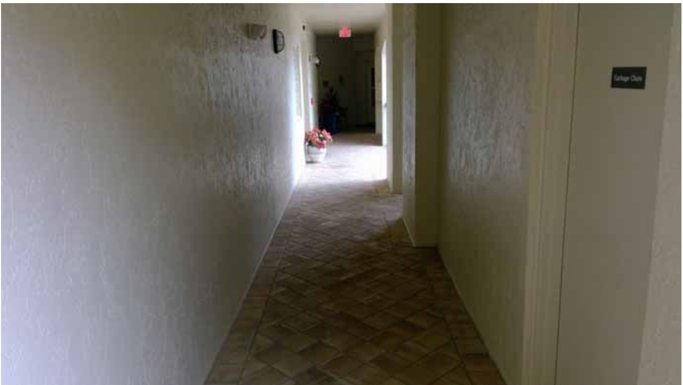
Building D Common Walkway - Upper Floor
