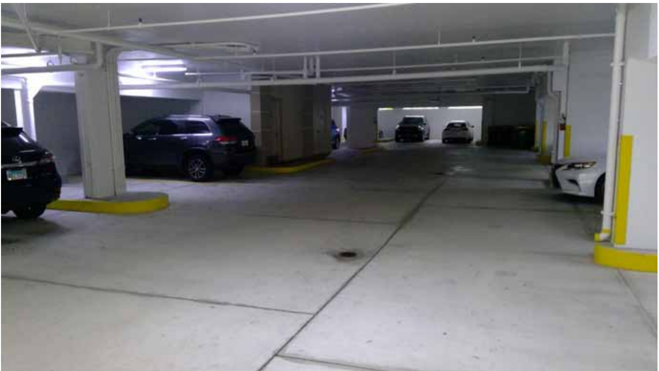
Building H Garage Level
