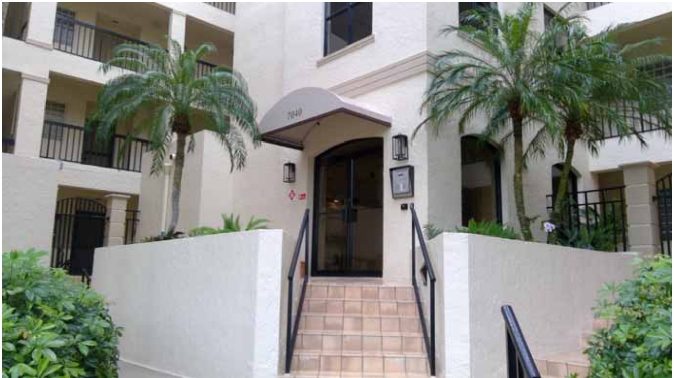
Building D Main Entrance
