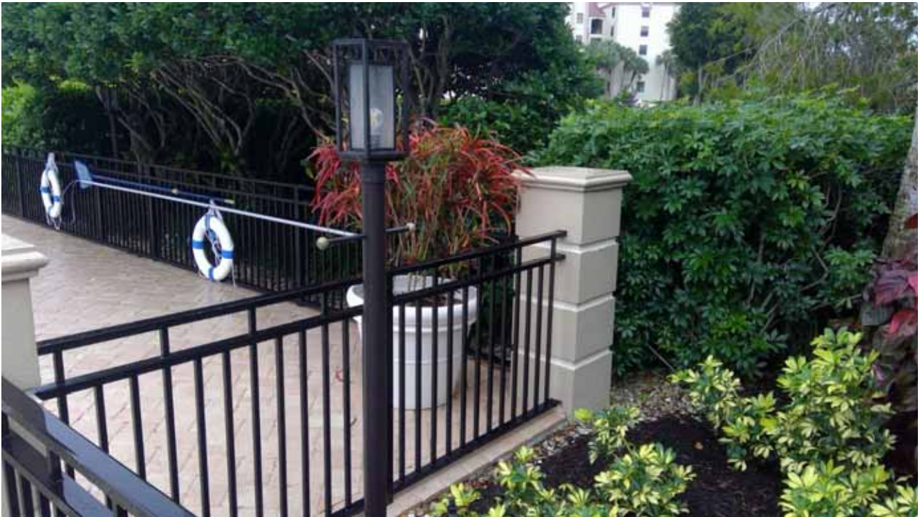
Light Pole & Fixture - Pool Area
