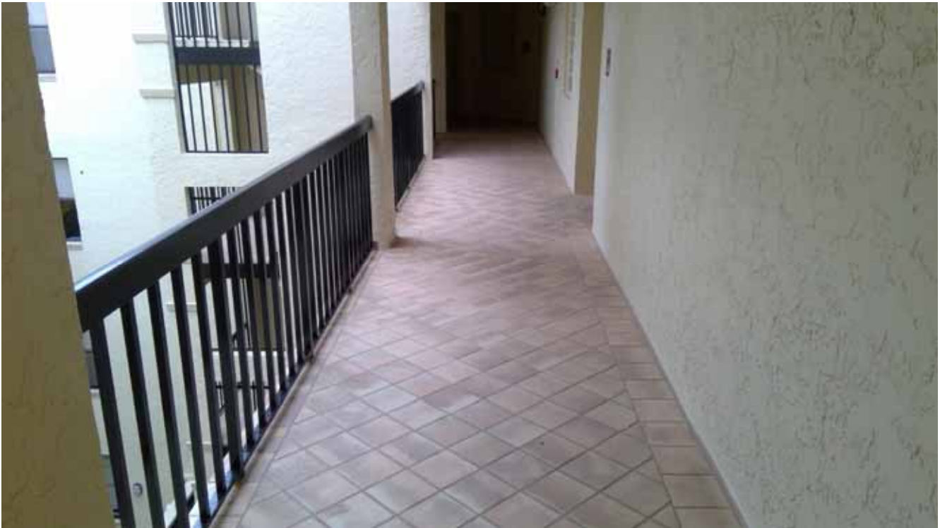
Building H Common Walkway - Upper Floor
