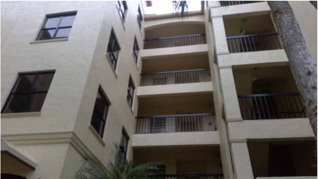
Building F Common Walkway & Railings
