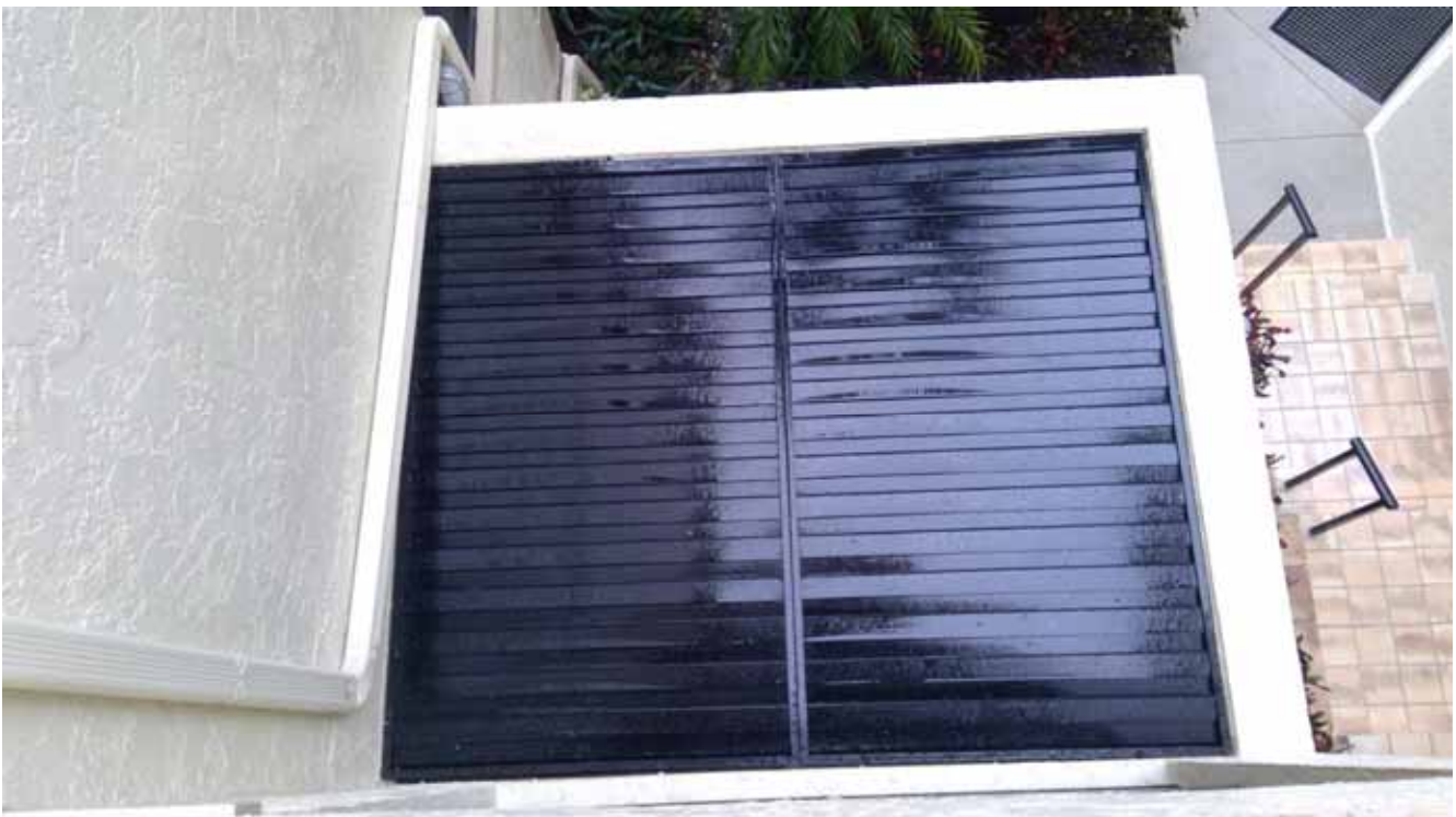
Building F Roof - Flat
