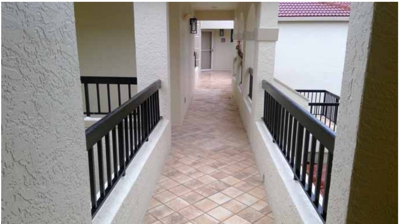
Building E Common Walkway
