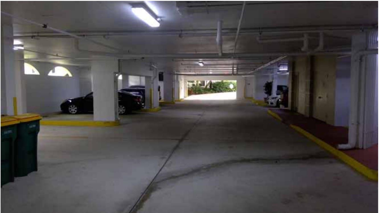
Building D Garage Level
