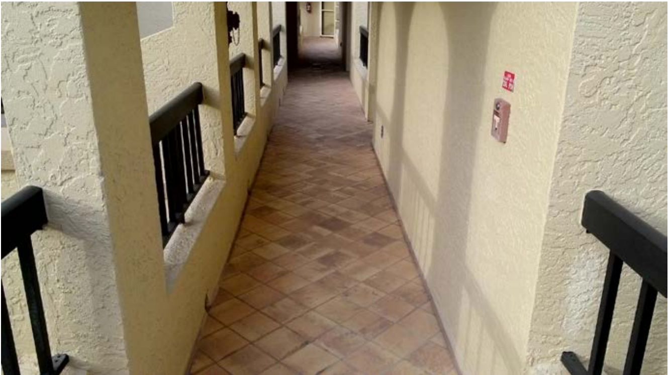
Building E Common Walkway
