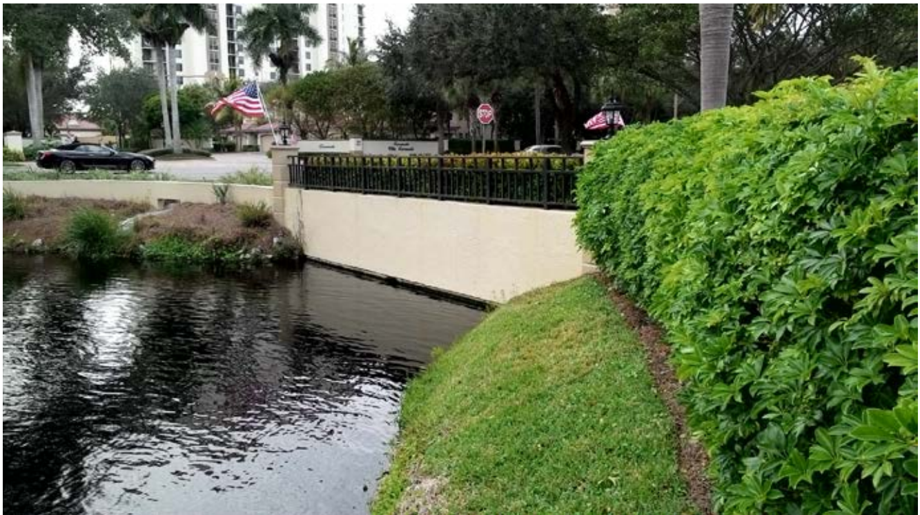
Entry Sidewall and Rail (1 of 2)
