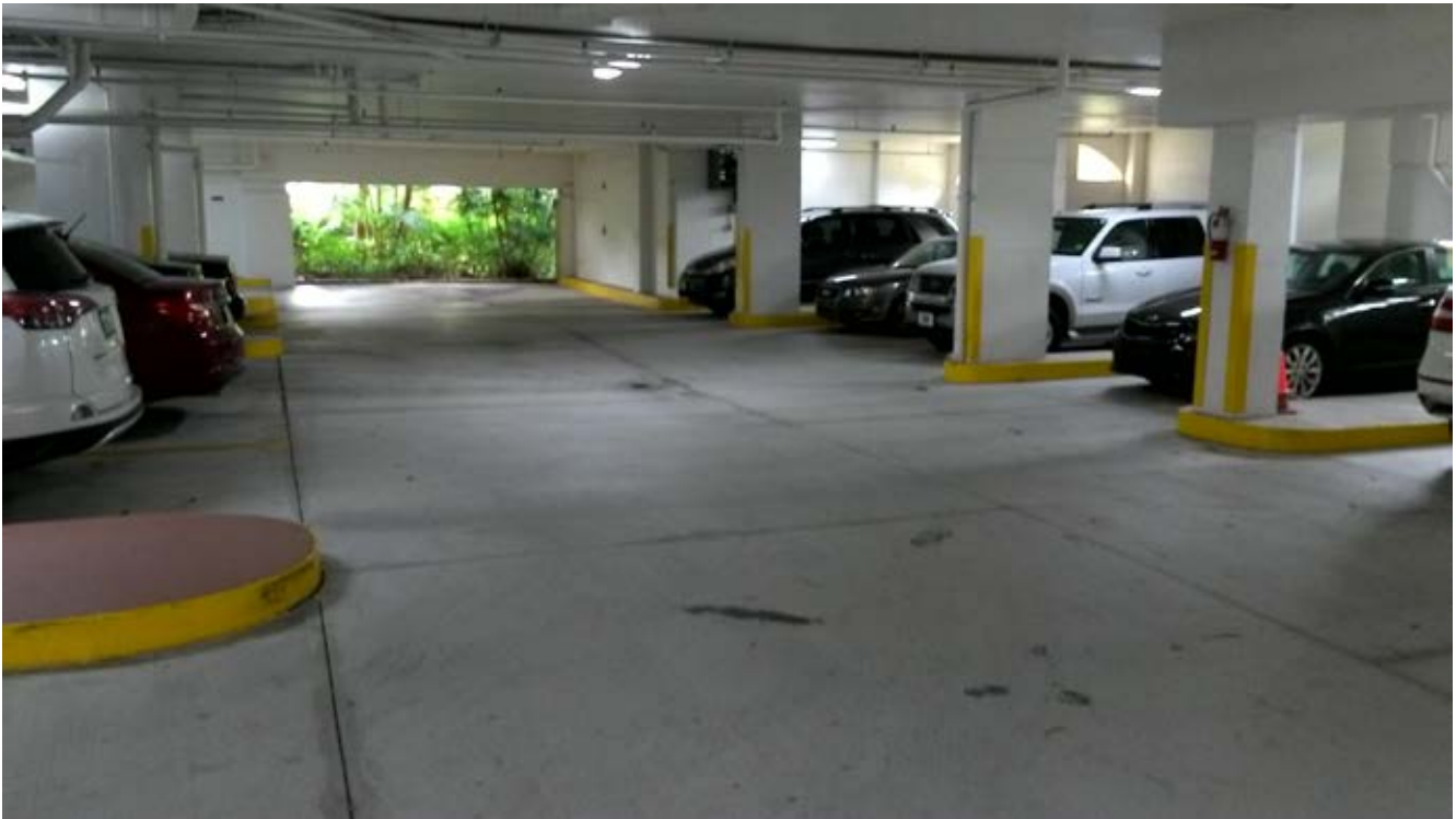
Building H Garage Level
