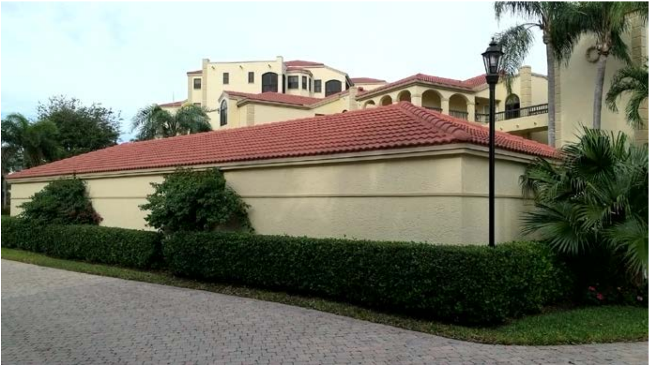
Building E Garage
