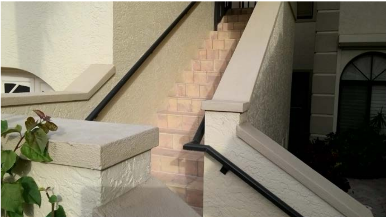
Building E Stairway
