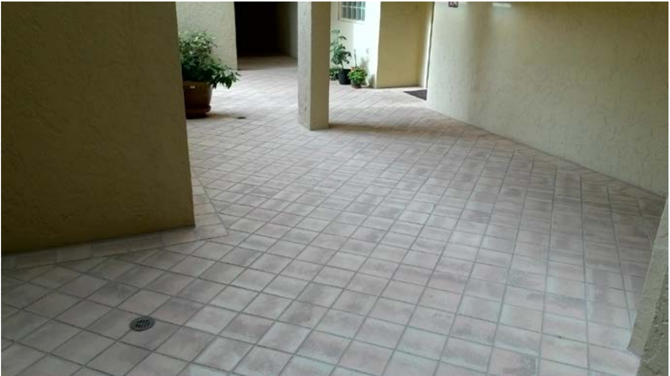
Building D Common Walkway
