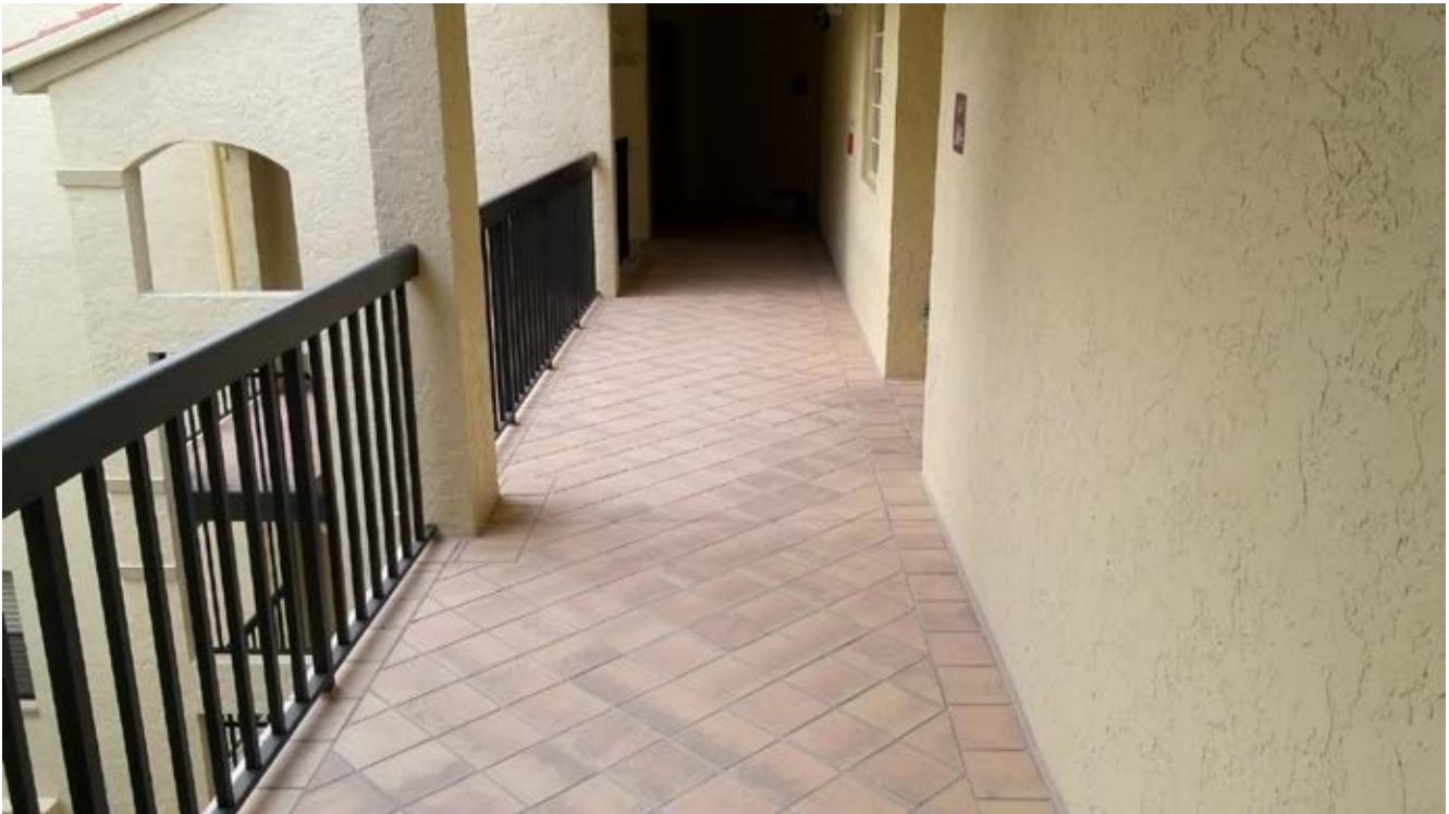
Building F Common Walkway
