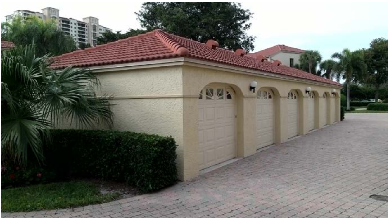
Building E Garage
