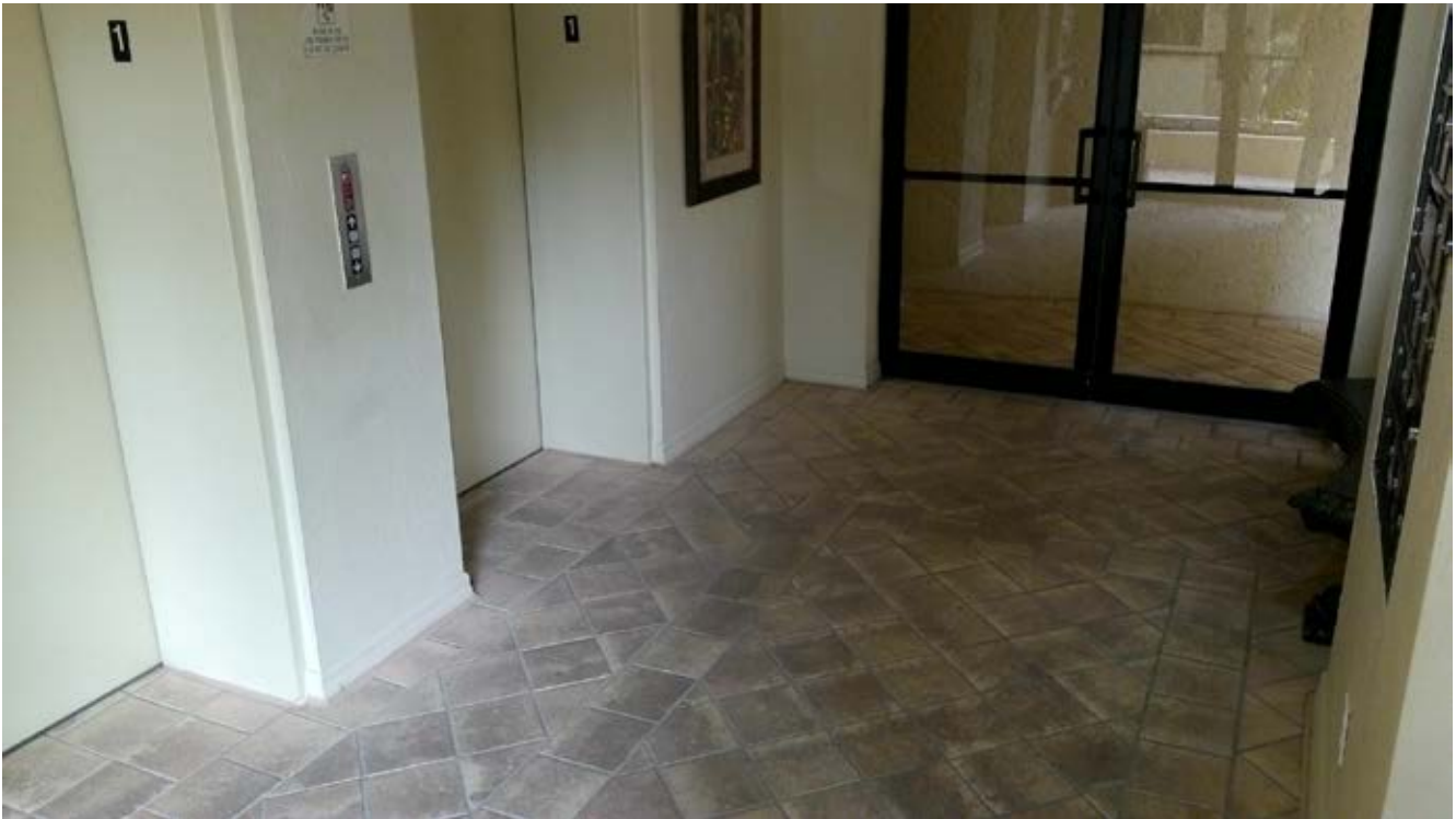
Building H Elevator Lobby - First Floor
