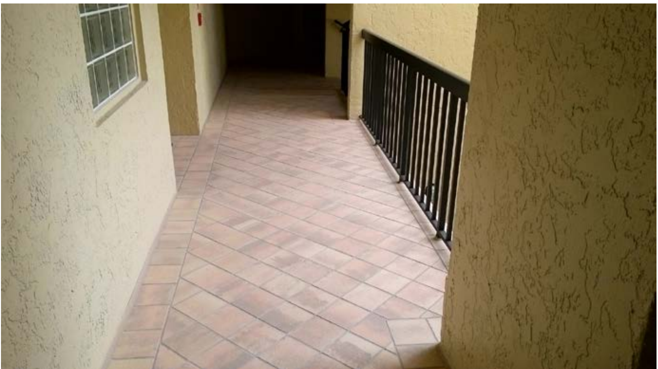
Building D Common Walkway
