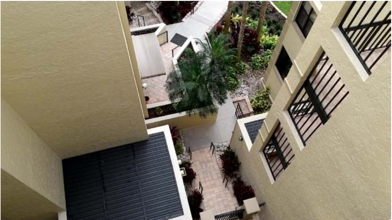
Building F Lower Level
