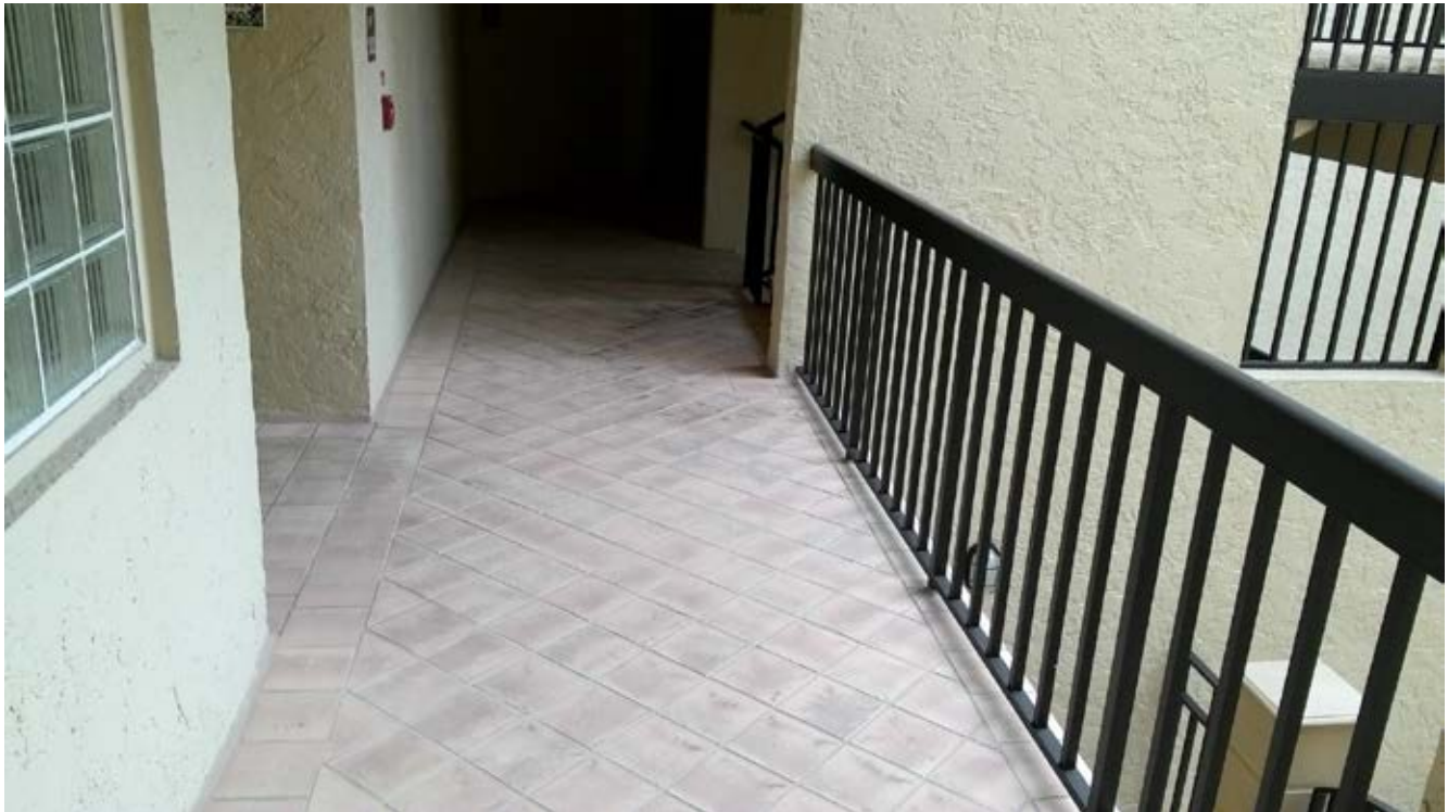
Building H Common Walkway - Upper Floor
