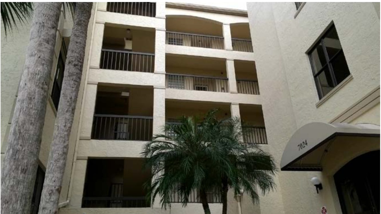
Building F Common Walkway and Railings
