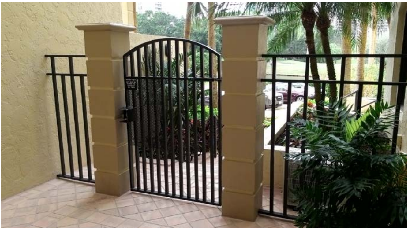
Building D Entry Gate
