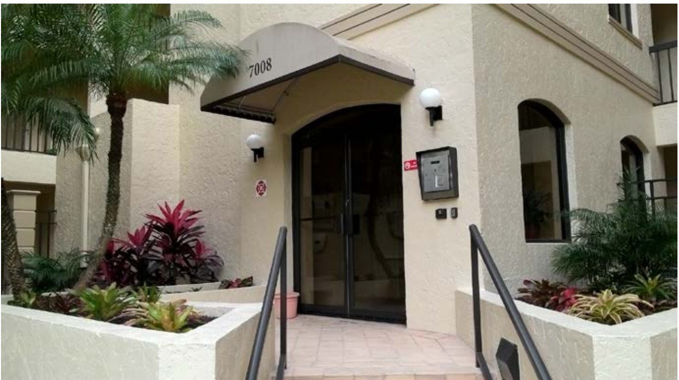
Building H Main Entrance
