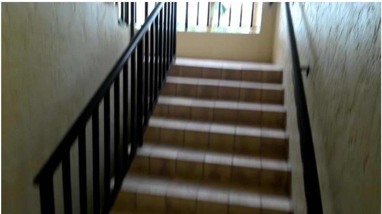
Building D Stairway
