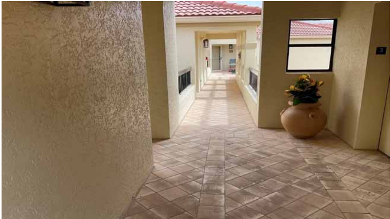
Building C Walkway - Upper Floor
