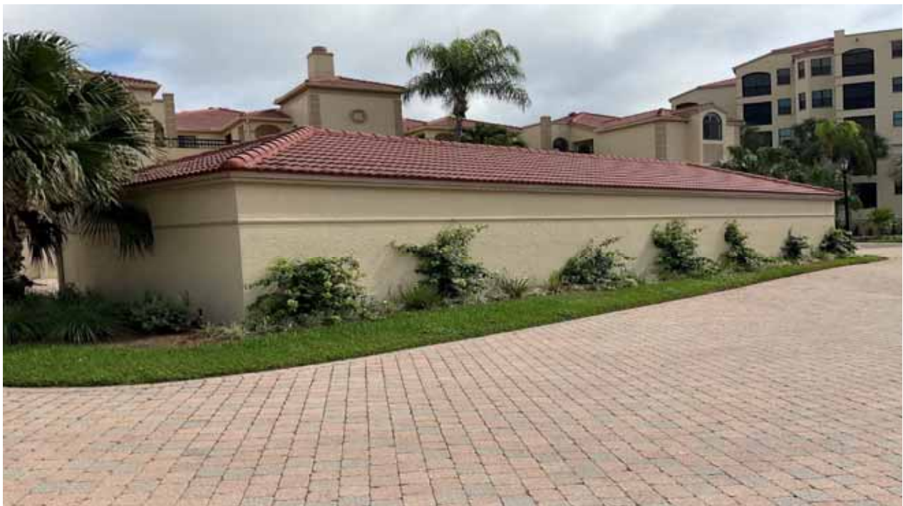
Garage, 6 Car (Bldg E)
