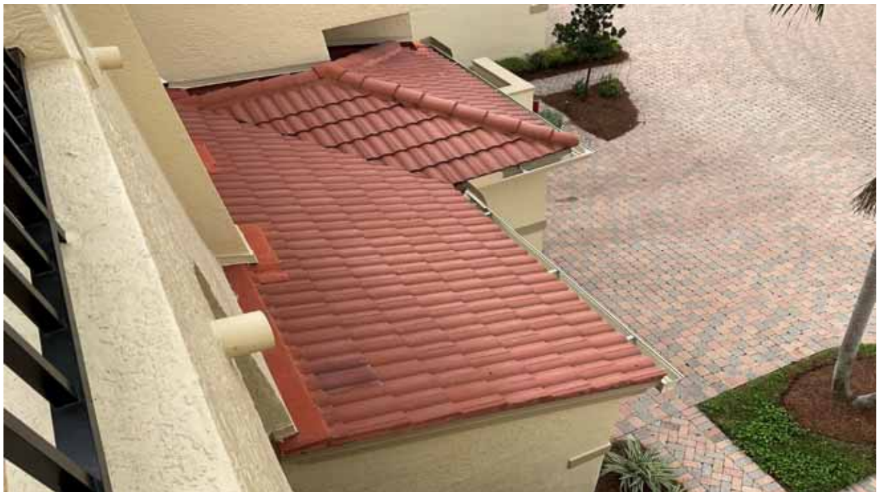
Building E Roof - Lower
