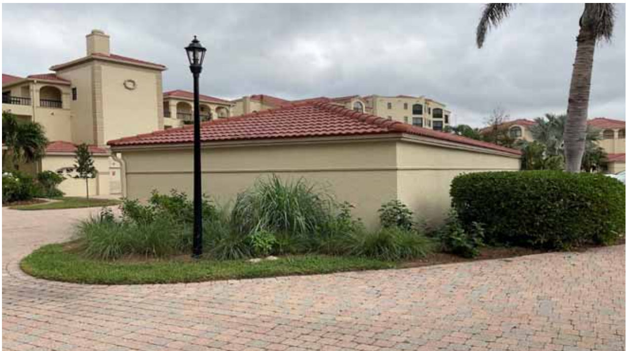
Garage, 6 Car (Bldg C)
