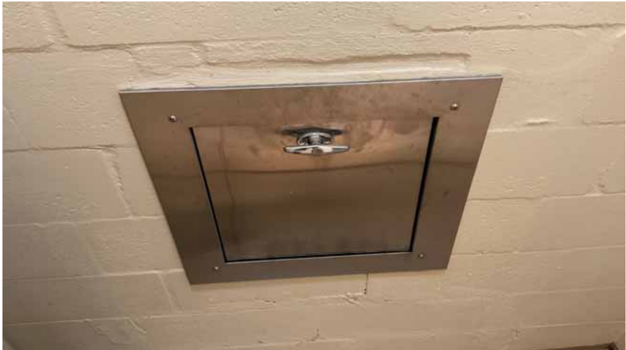
Building D Trash Chute Door
