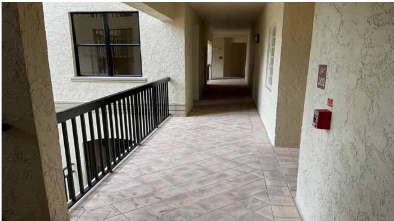
Building H Walkway - Upper Floor
