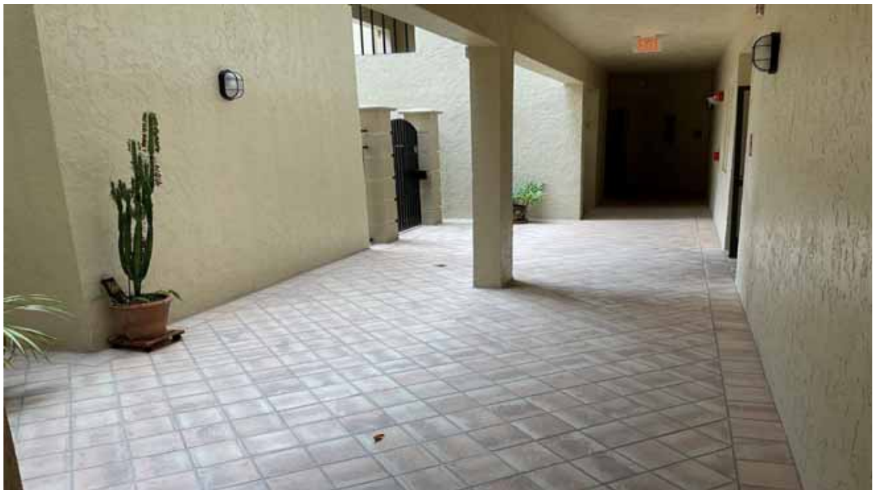
Building D Walkway - First Floor
