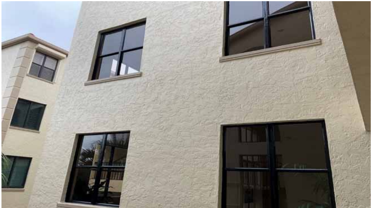
Building F Elevator Lobby Windows - Upper Floor
