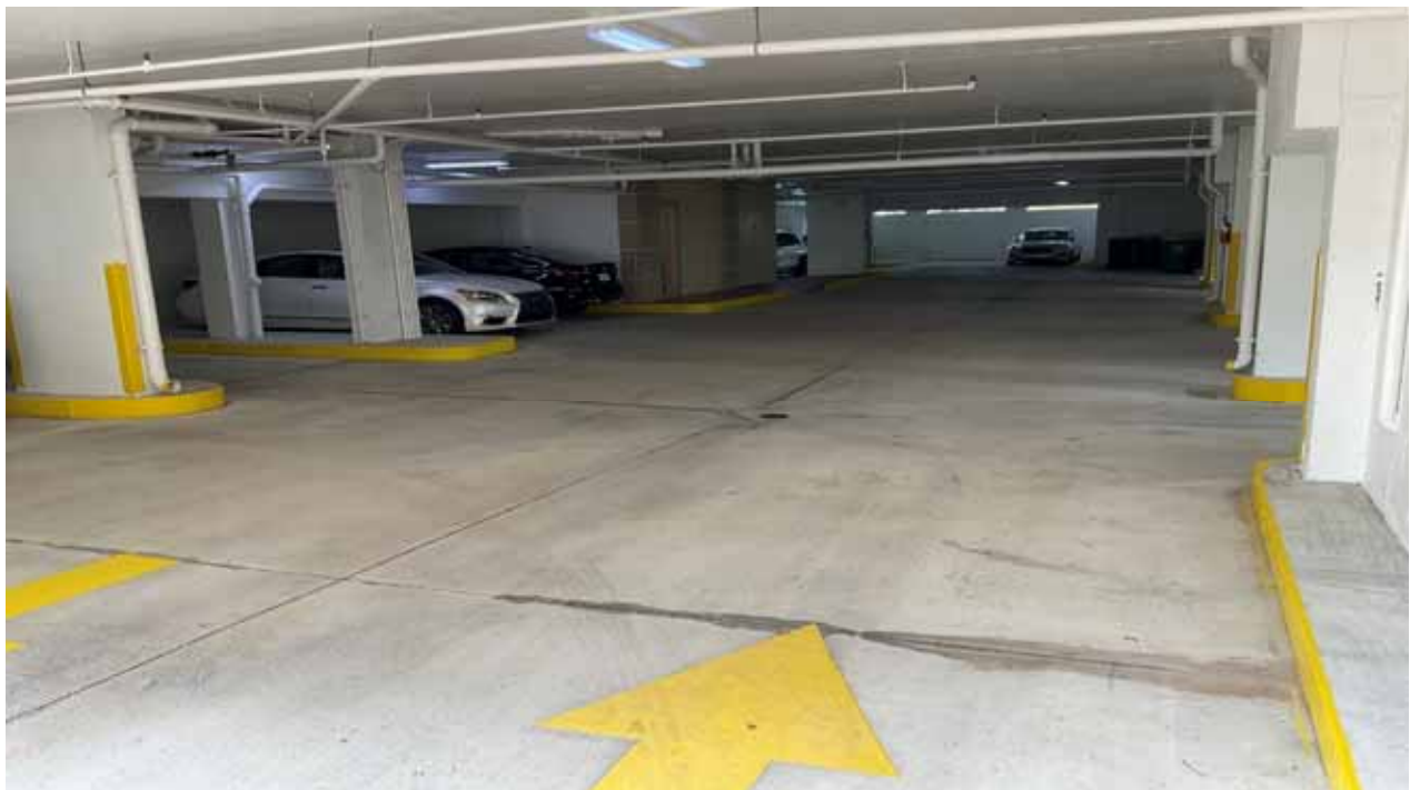
Building D Garage
