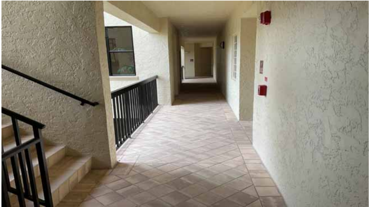
Building F Walkway Railing
