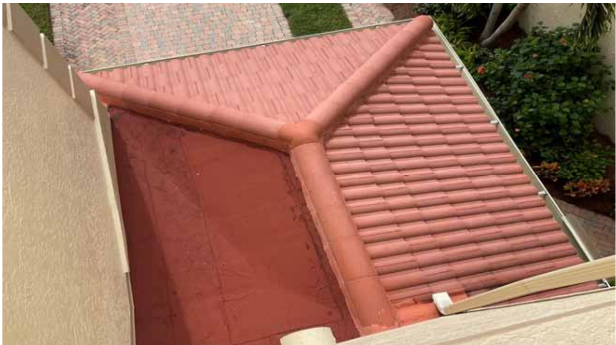
Building C Roof - Lower
