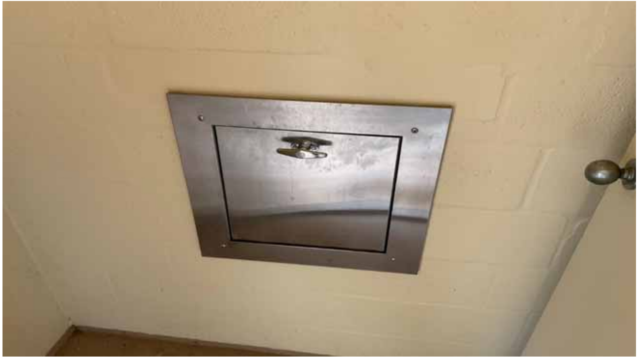
Building E Trash Chute Door
