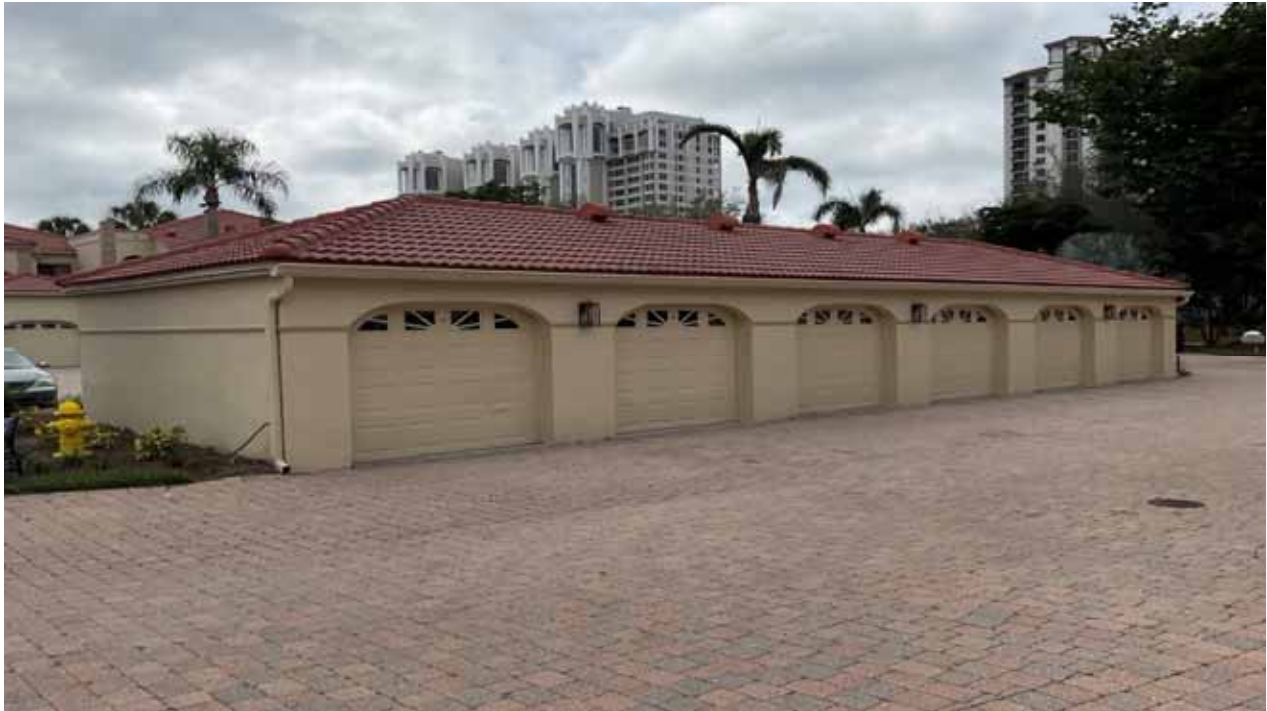
Garage, 6 Car (Bldg C)
