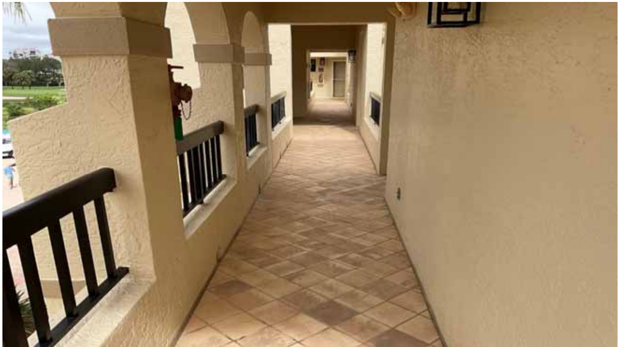
Building E Walkway - Upper Floor
