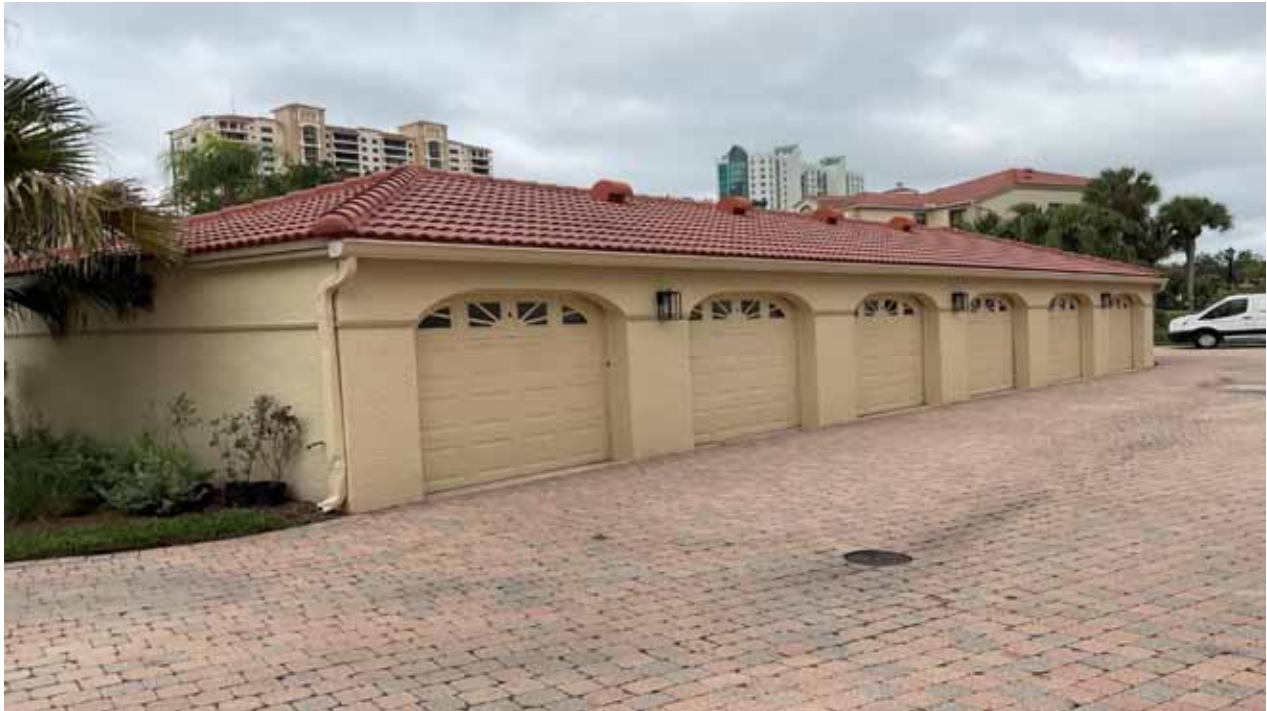
Garage, 6 Car (Bldg E)
