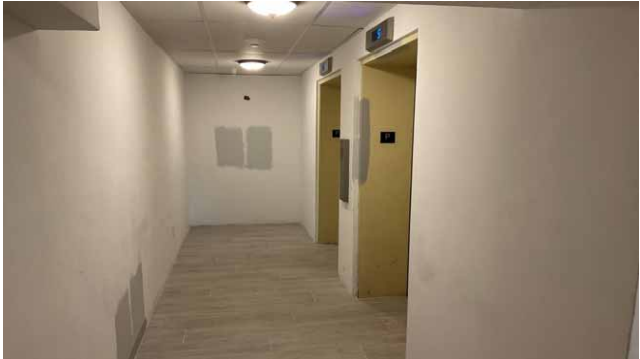
Building D Elevator Lobby - Garage
