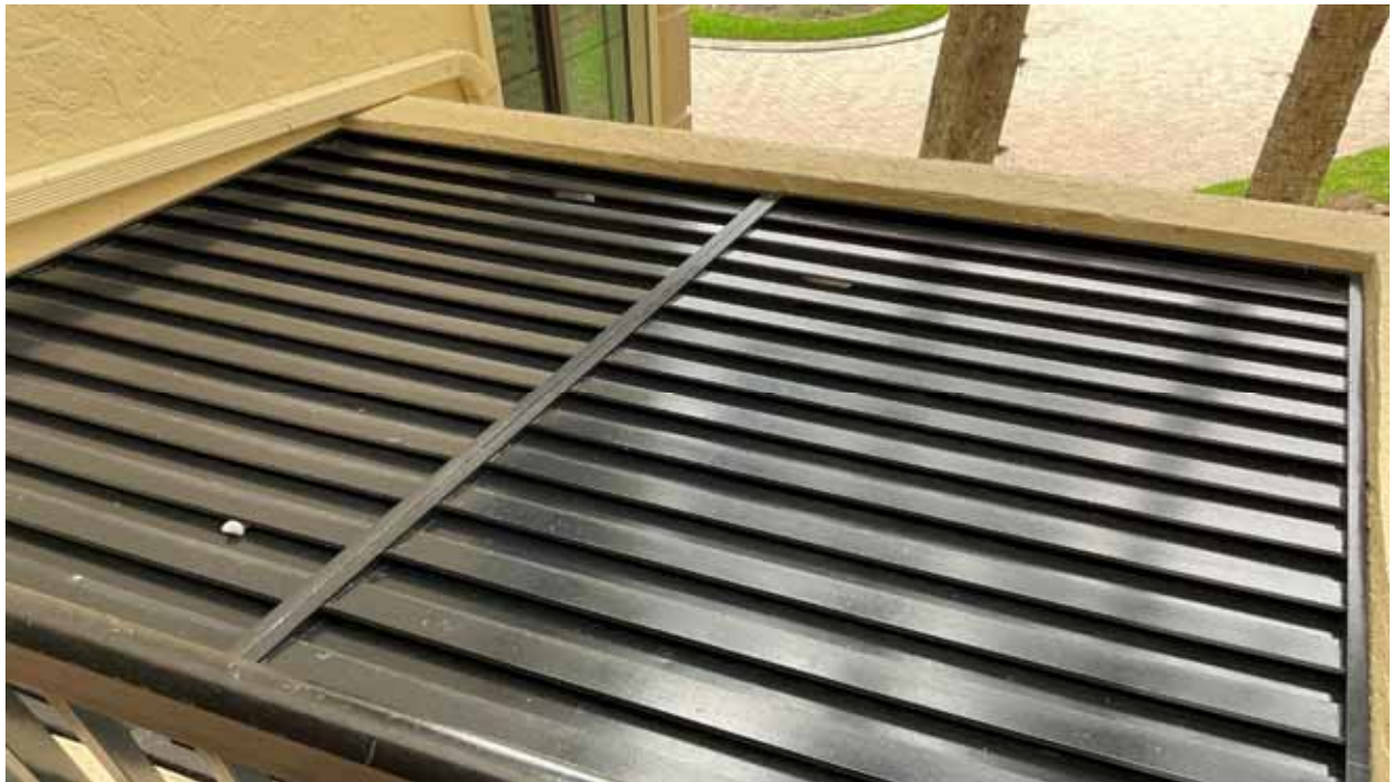
Building H Roof - Pump Room
