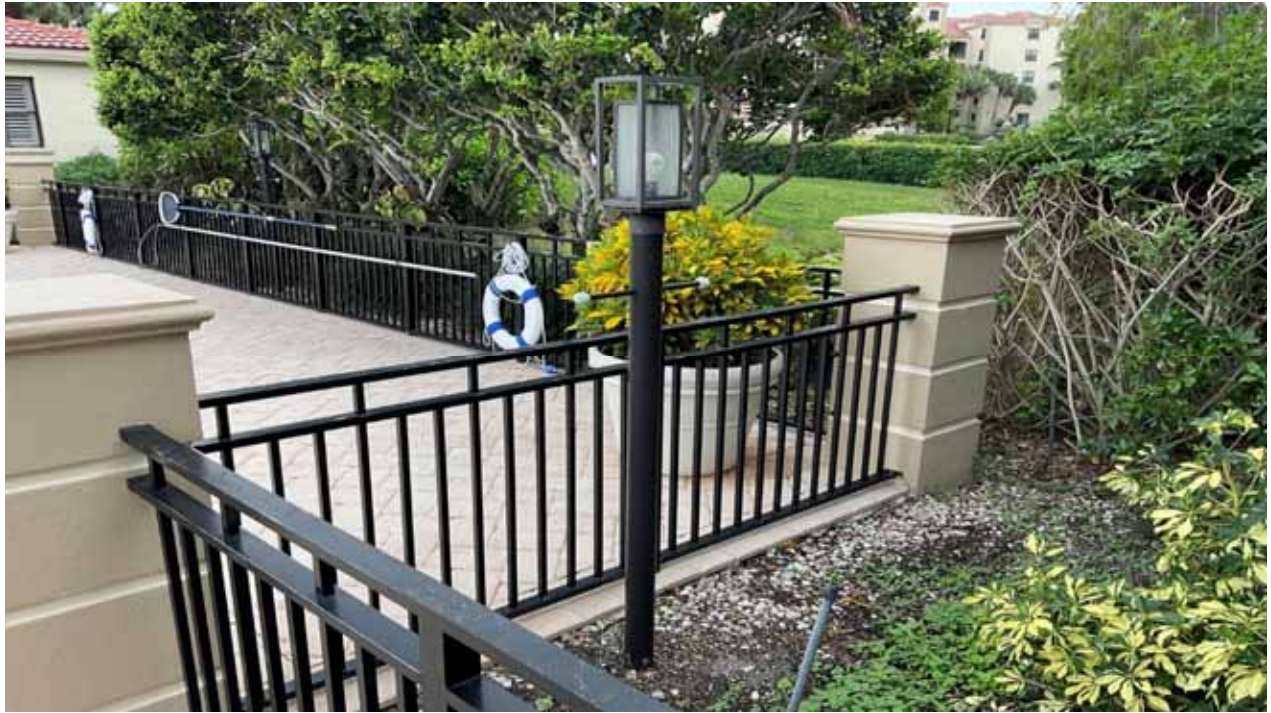
Light Pole & Fixture - Pool Area
