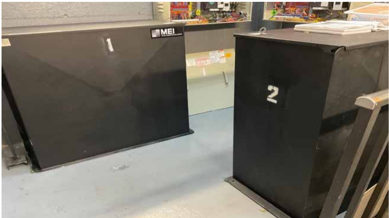
Building H Elevator Equipment
