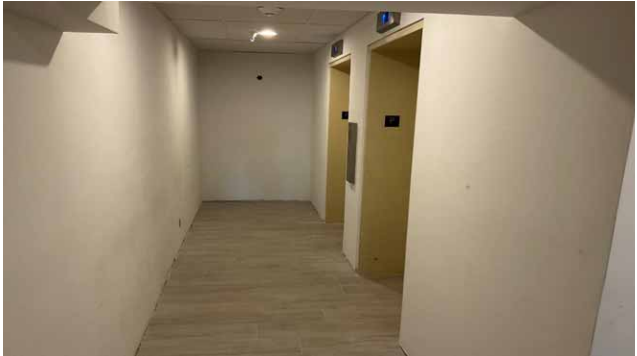
Building F Elevator Lobby - Garage
