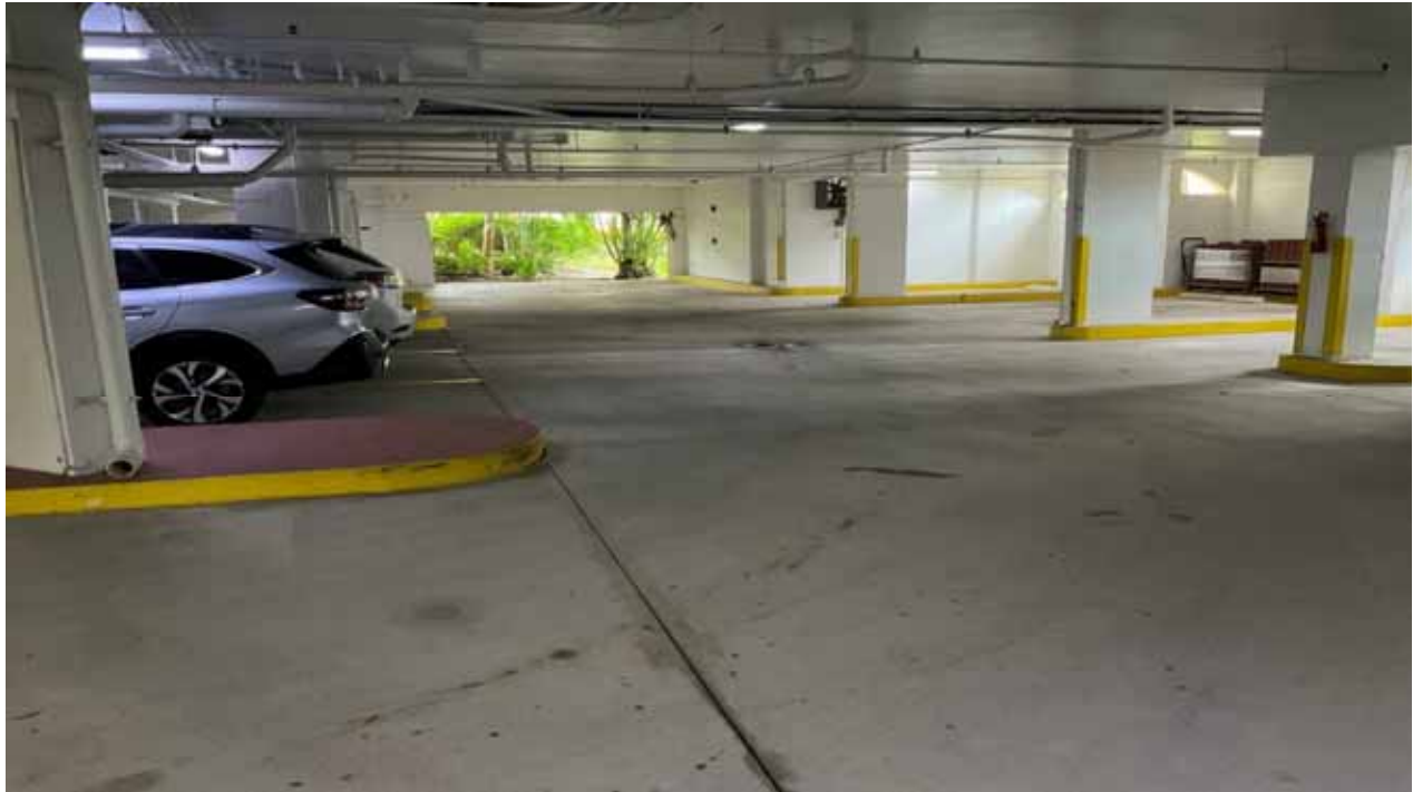
Building H Garage
