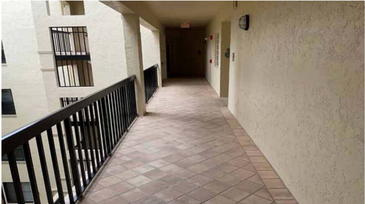
Building D Walkway - Upper Floor
