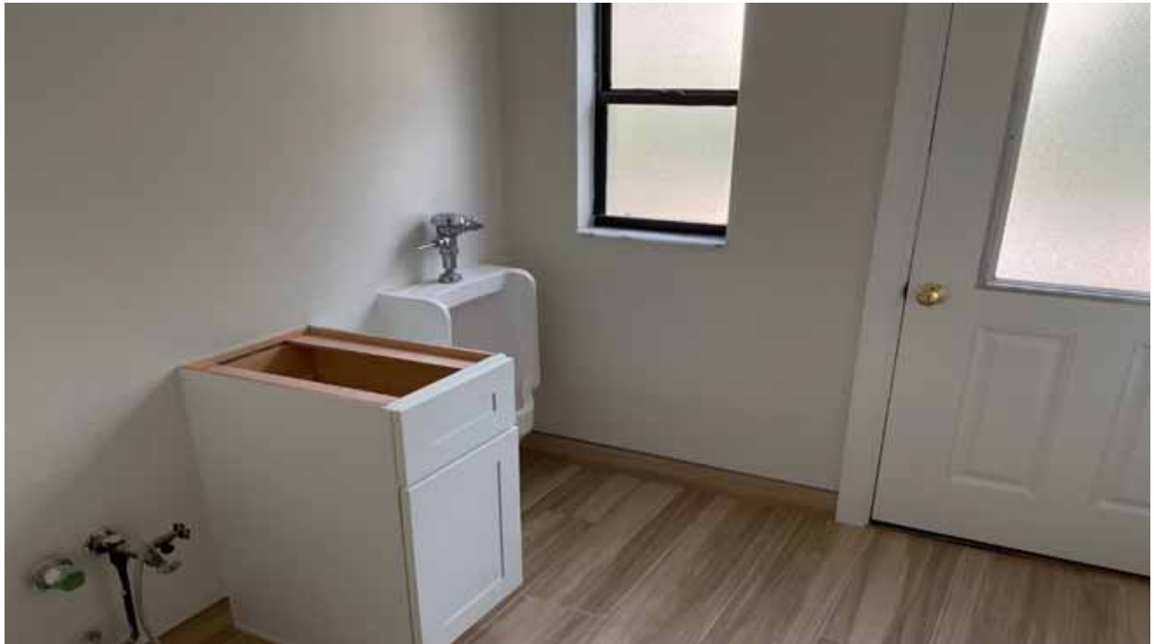
Clubhouse Restroom, Men's
