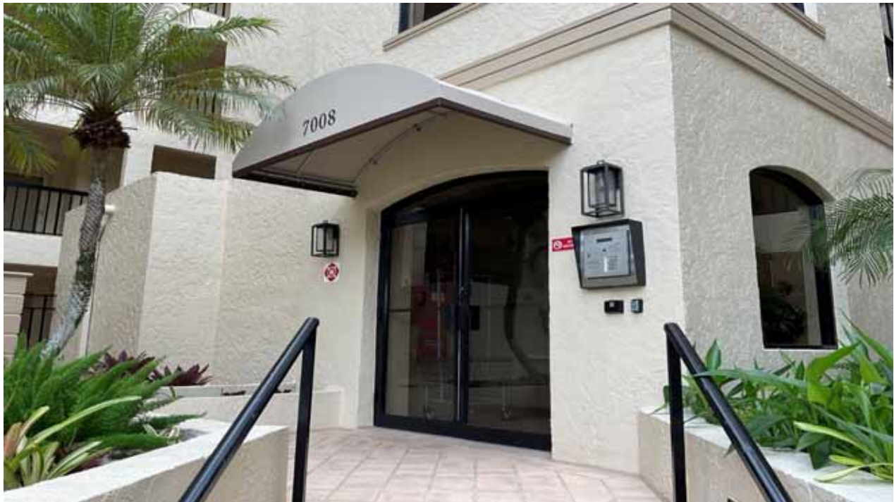
Building H Main Entrance
