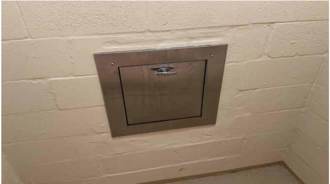
Building F Trash Chute Door
