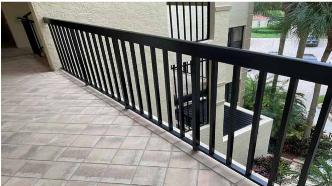
Building F Walkway - Upper Floor
